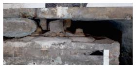
Photo-1 Damaged shoes found in a Gerber hinge
