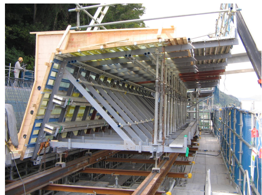
写真-4 送り出し型枠
