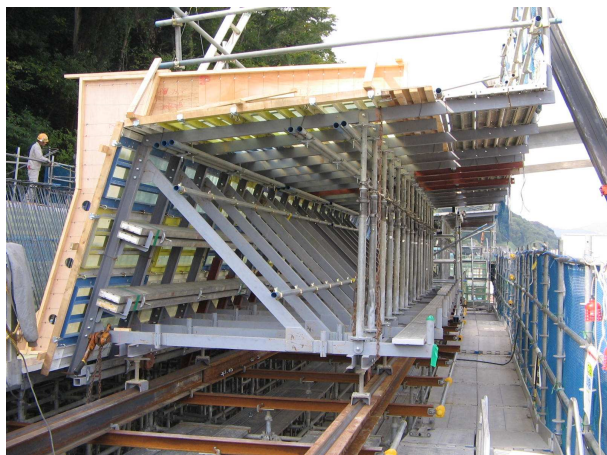
写真-9 送り出し型枠
