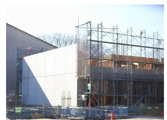
写真-7 棟間妻壁
